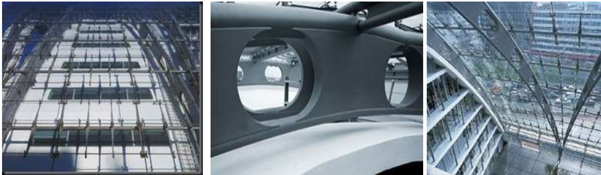
Figure 2.0.1.8. Berliner Bogen Office Building
